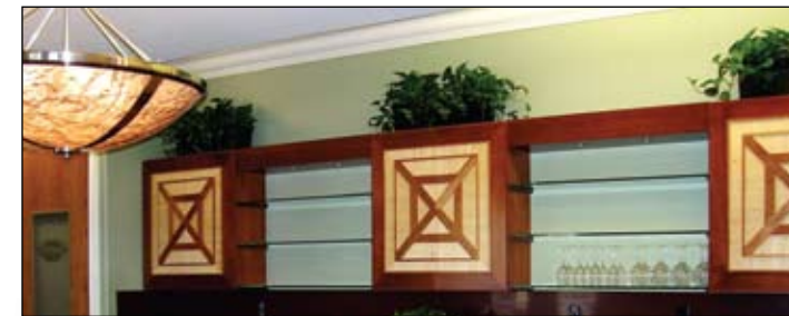
Board room cabinetry uses bamboo inlay on touch-latch doors. See the development from line drawing to finished installation.
